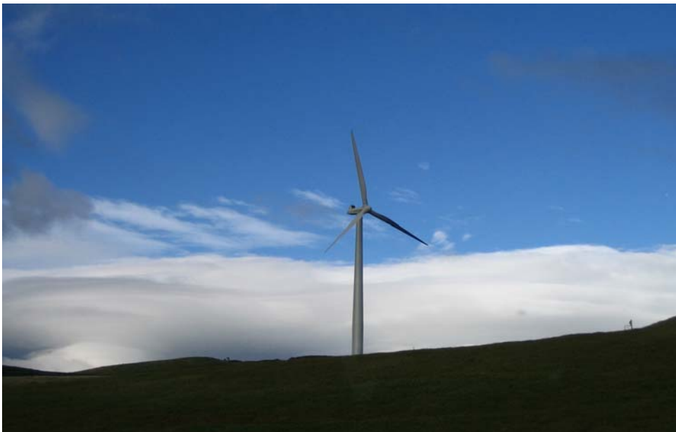
Wind farm at Wanganui
