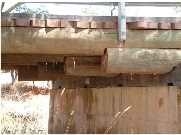
Figure 2 Close-up photo of the tested bridge
