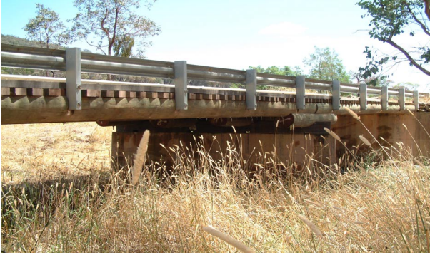
Figure 1 Photo of the tested bridge
