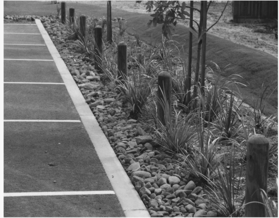
Figure 4: - Infiltration Trench Adjacent to Public Carpark
