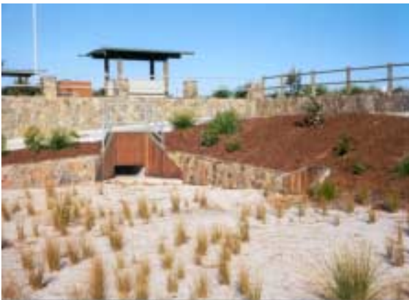
Figure 5: - Isolated Infiltration Basin in Central Precinct
