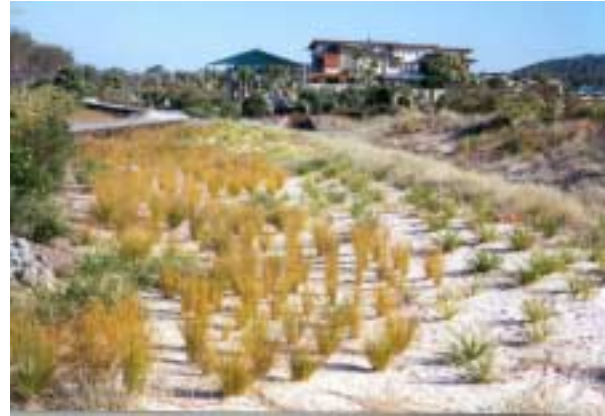
Figure 6: - Infiltration Basin in Frontal Swale. (Note the boardwalk has been integrated into the swale area)
