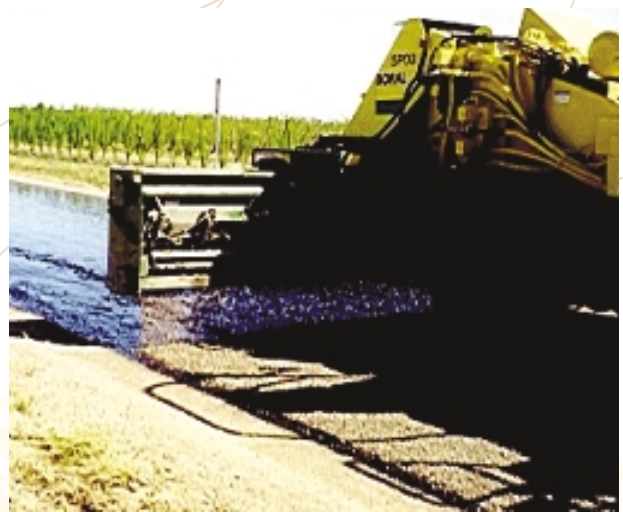
Figure 4. GATT aggregate spreader
