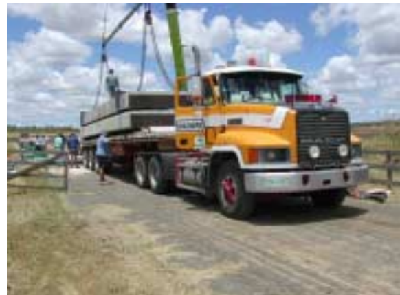
Figure 6 Transportation of bridge sections
