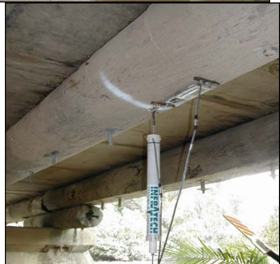
Figure 7 Test truck crossing bridge instrumented to measure deflection and strains.
