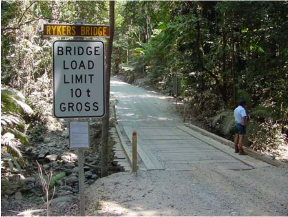
Figure 4 This load limited bridge has been replaced.
