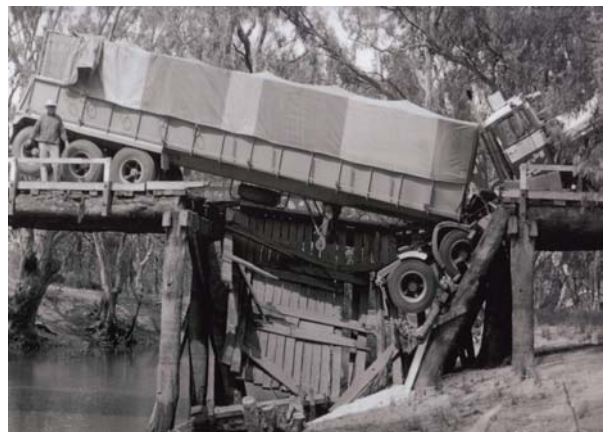
Figure 1 Failure of a timber bridge under load (interstate location).
