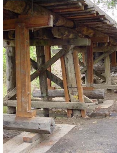
Figure 5 Temporary piers to strengthen deteriorated girders
