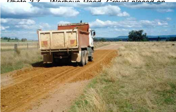
Photo 3.7 – Warboys Road. Gravel placed on
