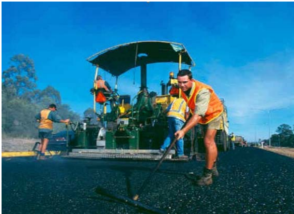
Figure 7. Laying hot-mix asphalt
