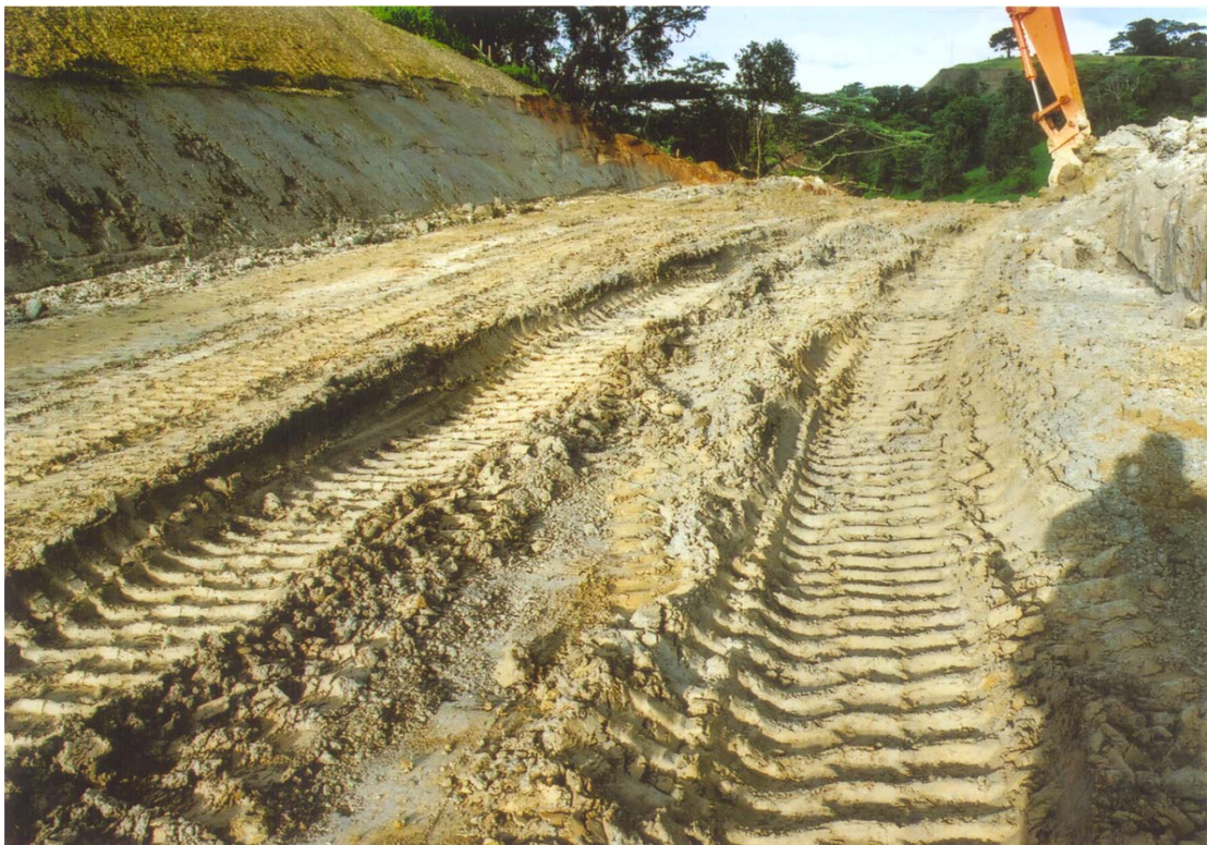
Cutting Subgrade
