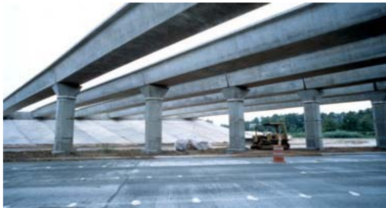
Precast Concrete Tub Girders in Place
