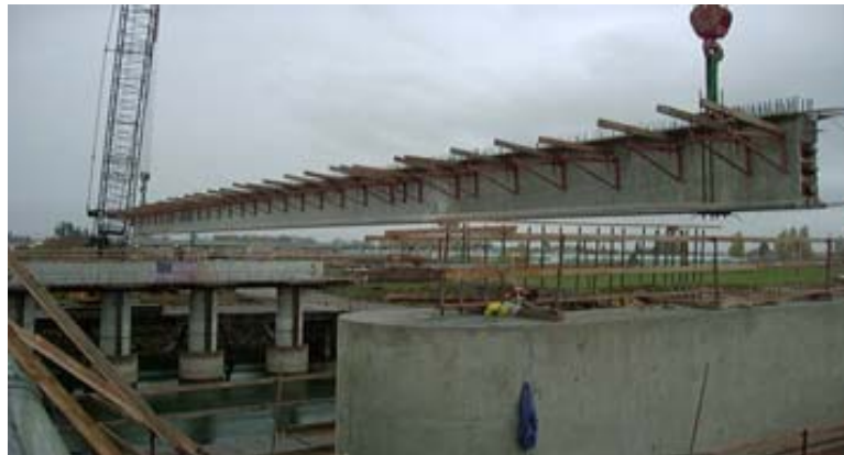
Spliced Girder Being Placed
