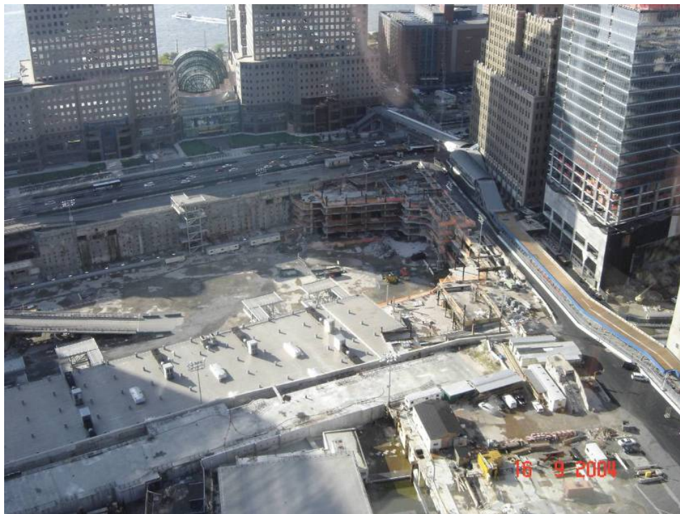
World Trade Centre Site under Reconstruction
