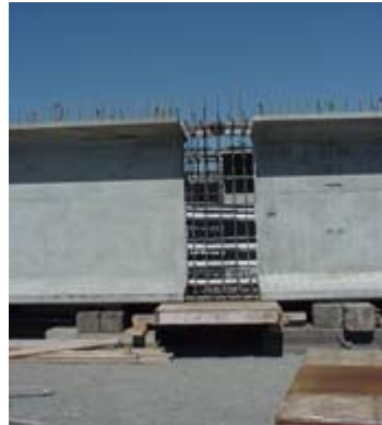
Girder Being Spliced On-Site
