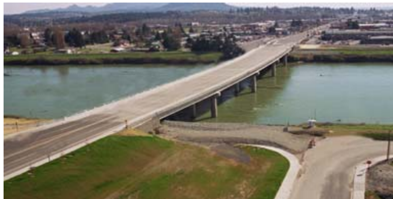
Completed Riverside Bridge over Sagit River, Washington
