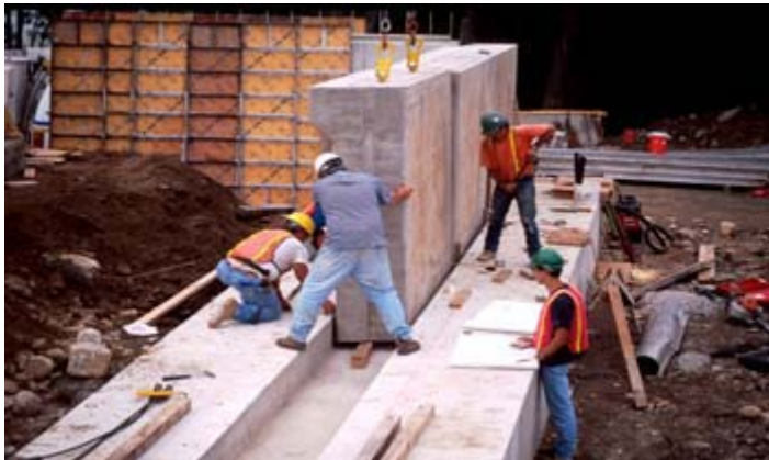
Precast Concrete Abutment
