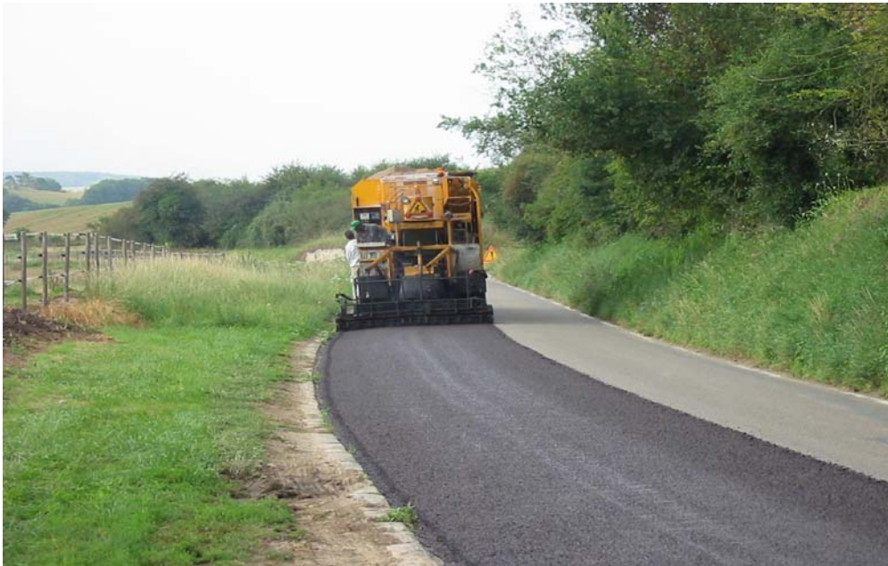
Image 009 – Application of Gripfibre on rural road
